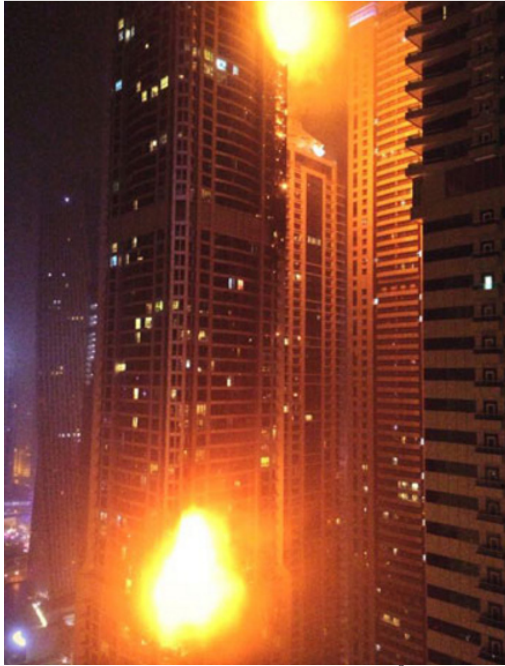
(23. 2. 2015: Torch-Tower in Dubai. 5 )
